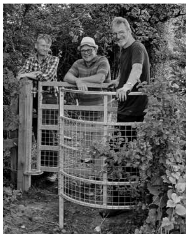
Men's Shed members are pictured after installing one of the two new gates near Middle Stoughton.
