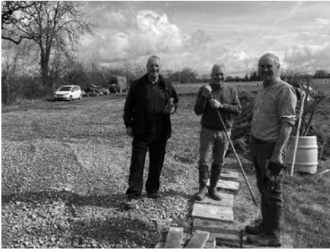
Members helping to lay the new car park.
