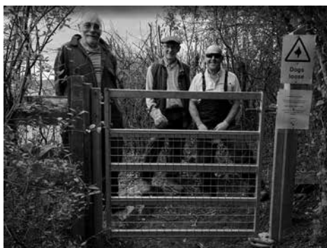
Yet another gate gets installed!
